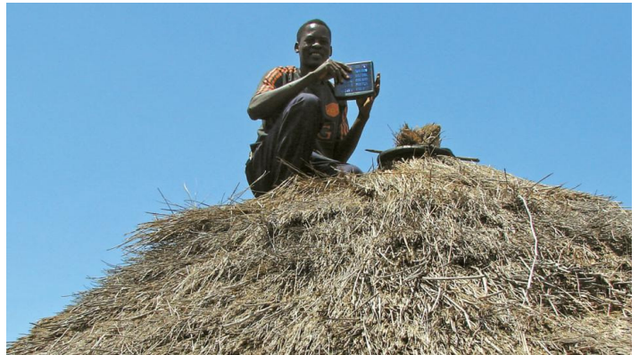
A young man installs a solar panel on a thatched roof, which when connected to solar lights inside the hut, will extend the villagers' day by three to four hours.
