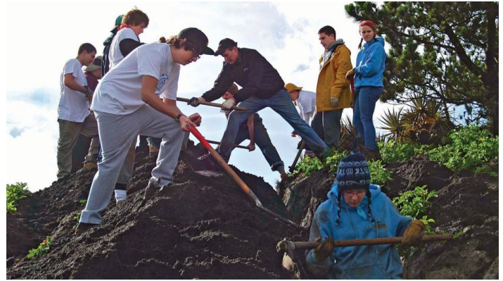
High school students from the Builders Beyond Borders program help install pipes that will carry water to the mountain town.
