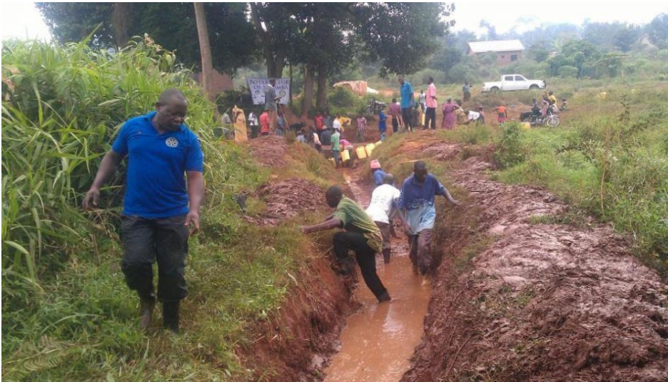
Members of the Rotary Club of Nkumba, Uganda, help to refurbish a water well, resulting in a 40 percent increase of water flow. Photo Credit: Courtesy of Michael Muriithi
