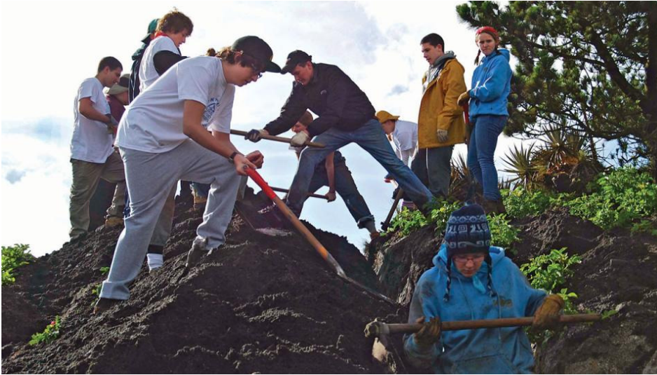
High school students from the Builders Beyond Borders program help install pipes that will carry water to the mountain town. Photo Credit: Photo by Tony Riggio
